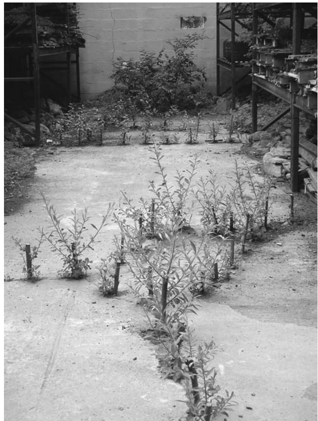
Figure 15. Transformer: parts of the concrete floor are drilled and planted ('Green dynamite'). ©Rumelhart.
