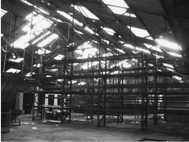
Figure 12. Transformer: racks filled with a mixture of waste wood and soil as 'Big Macs,' initial phase. ©Rumelhart.
