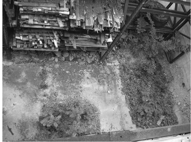
Figure 13. Transformer: racks filled with a mixture of waste wood and soil as 'Big Macs,' initial phase. ©Rumelhart.
