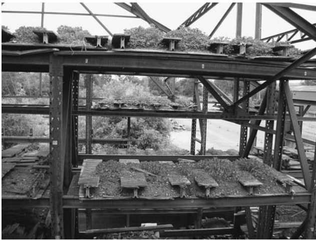
Figure 14. Transformer: succession of plants in the racks. ©Rumelhart.
